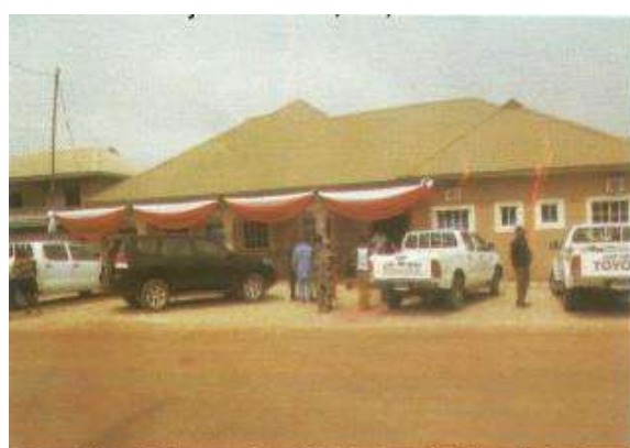
Completed Akpugo Health Centre Oji River L.G.A Project Cost N9,970,600.00
